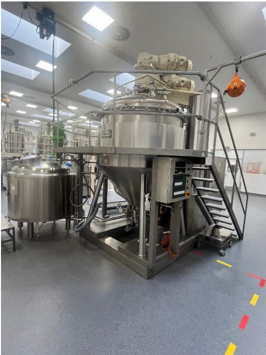
Complete production facility for creams
